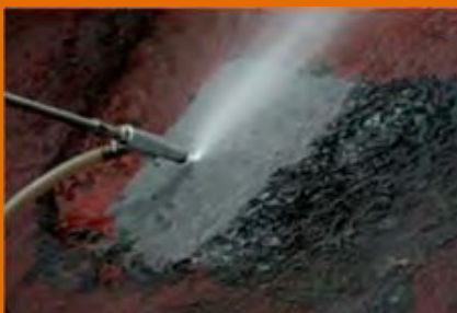
Surface sand blasting
